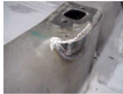
Here the welds are ground smooth.
