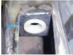
Bushing support tach welded in place.
